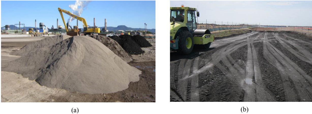
Figure 2: Compaction trial (a) Coal wash and steel furnace slag and (b) Vibration roller
