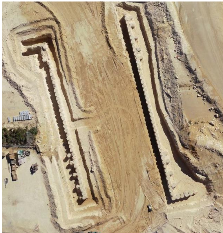
Figure 5: Bridge No.1 pile capping beam excavation
