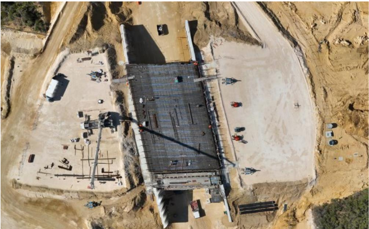
Figure 7: Bridge No.2 during construction
