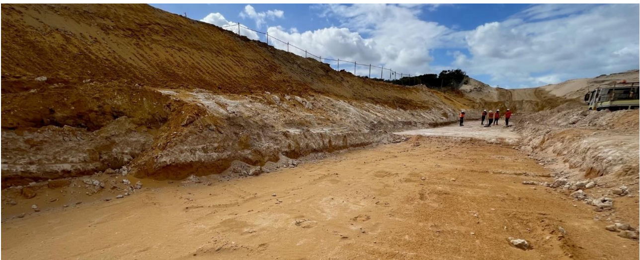
Figure 9: Bridge No.2 footing excavation (across sand / limestone interface)
