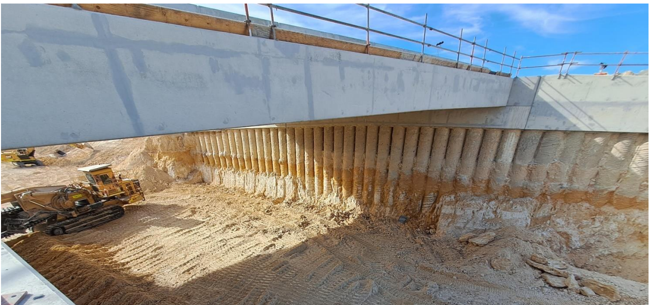
Figure 2: Bridge No.1 during bulk excavation works
