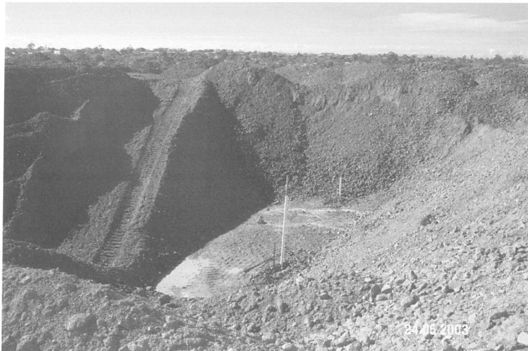
Figure 8 Upper and Lower Monitoring Plates with Temporary Type A Fill Stockpile
