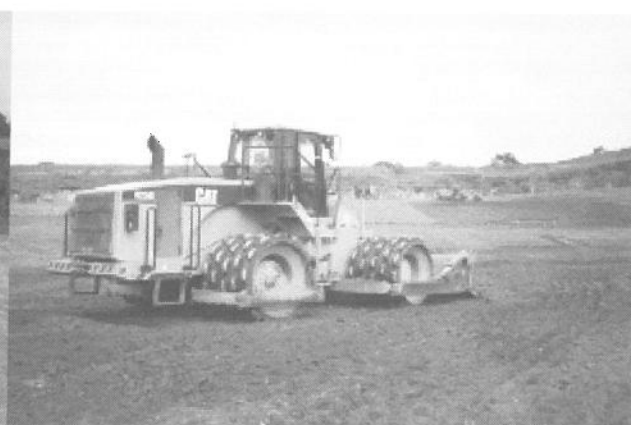
4b Fill Placement and Compaction
