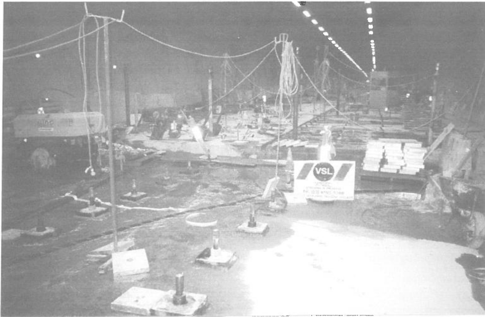
Photograph 3 – Twin anchored and multi-anchored slabs
