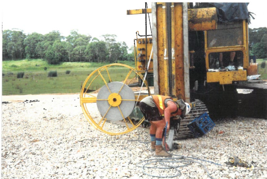
Photo 6: Close-up view of wick drainage rig
