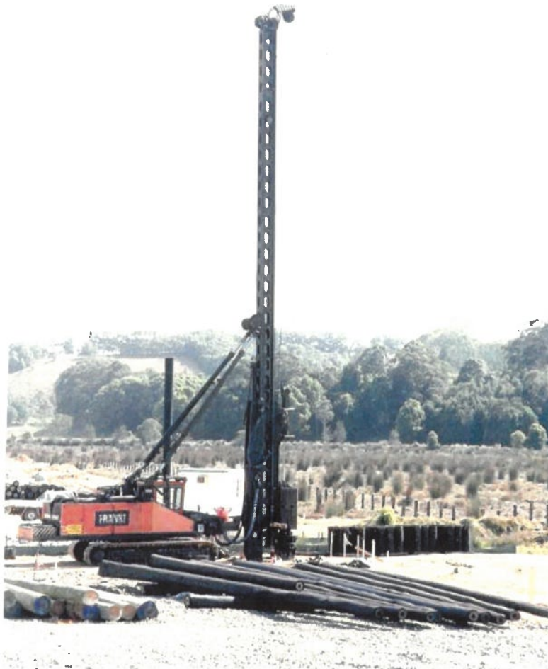
Photo 7: Installation of timber piles
