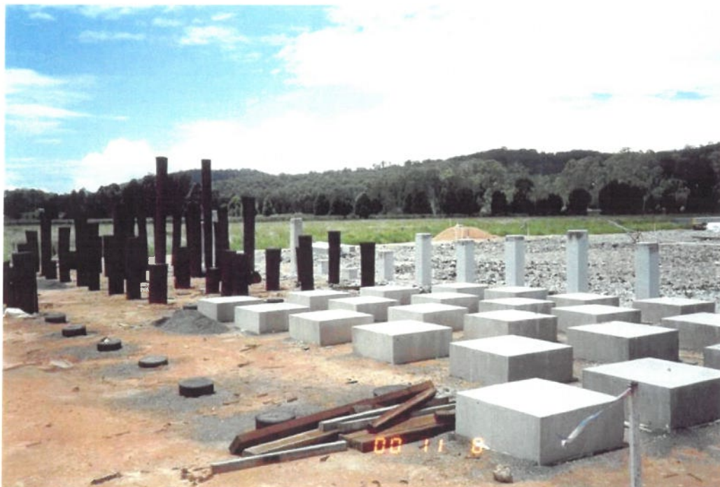
Photo 8: Constructed pile caps
