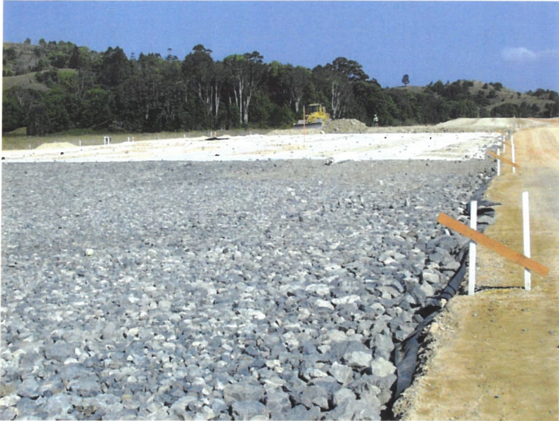
Photo 3: Placement of geotextile over drainage blanket
