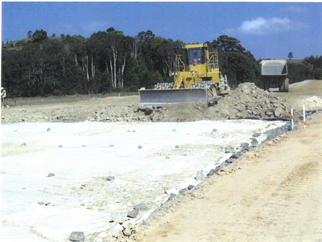
Photo 4: Placement of fill over geotextile
