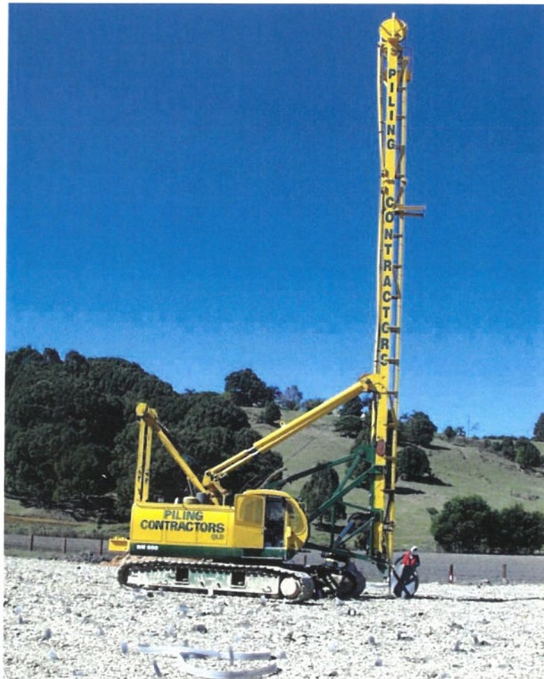
Photo 5: Installation of wick drains
