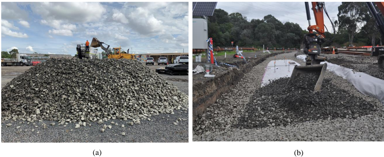
Figure 5: (a) Onsite blended RIBS (b) Placement of RIBS on track at reduced height ( 1 < \text{m} )
