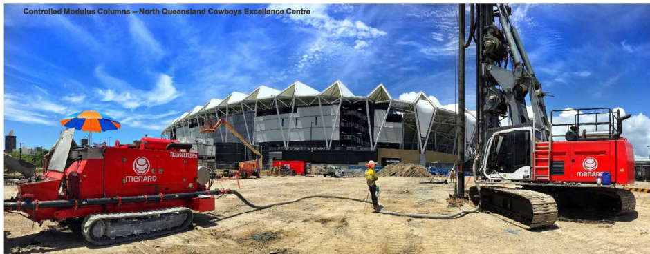
Controlled Modulus Columns – North Queensland Cowboys Excellence Centre
