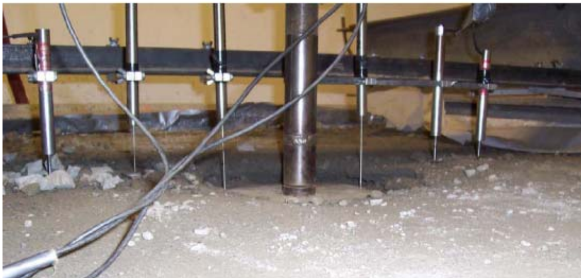
Load Plate and Displacement Transducer on aggregate surface
