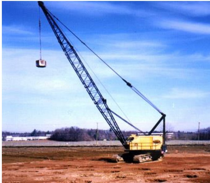
Deep Dynamic Compaction (DC)
