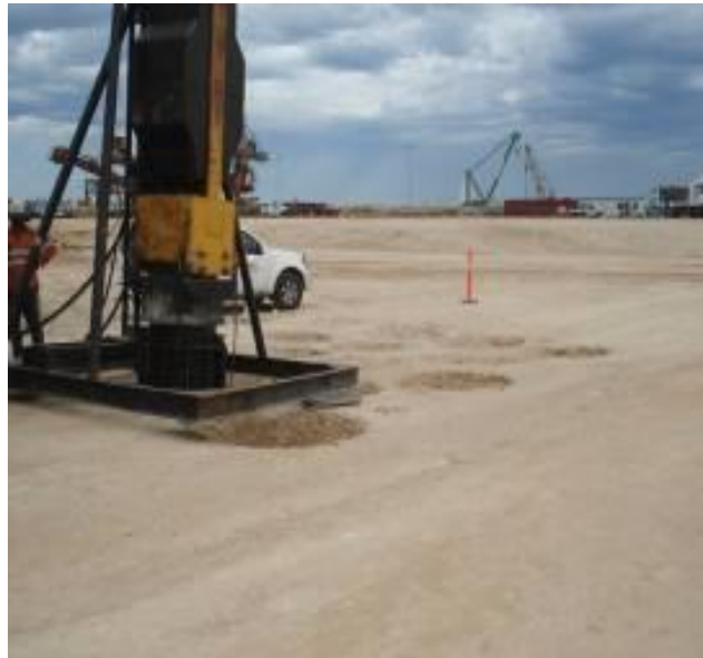
Rapid Impact Compaction (RIC/CDYC)
