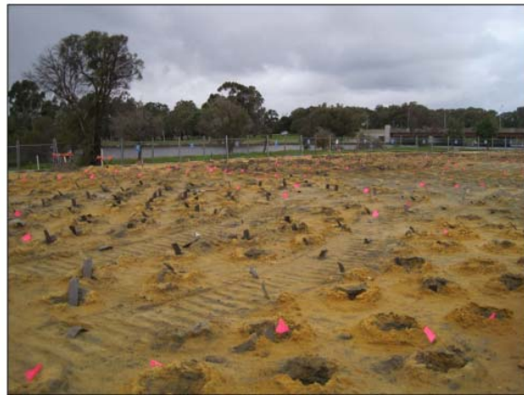
Plate 1: Wick drains along eastern edge of site (pink flag indicates auger refusal)
