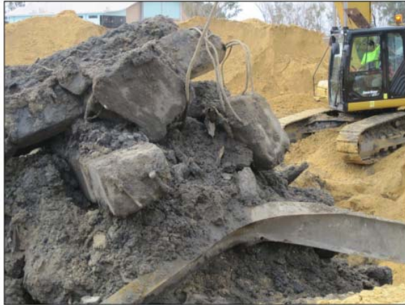
Plate 3: Obstructions found within old fill during Area C excavation (1)
