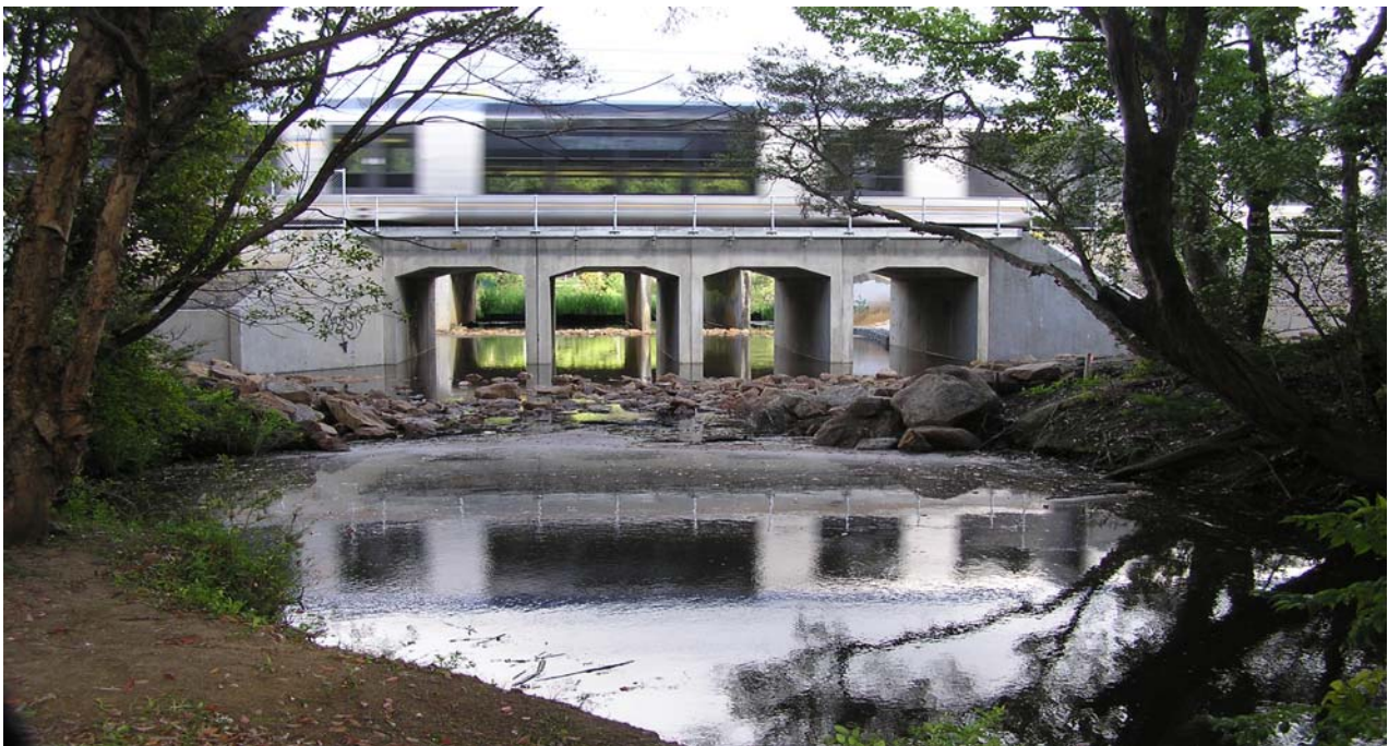
Figure 10: Completed rail bridge.
