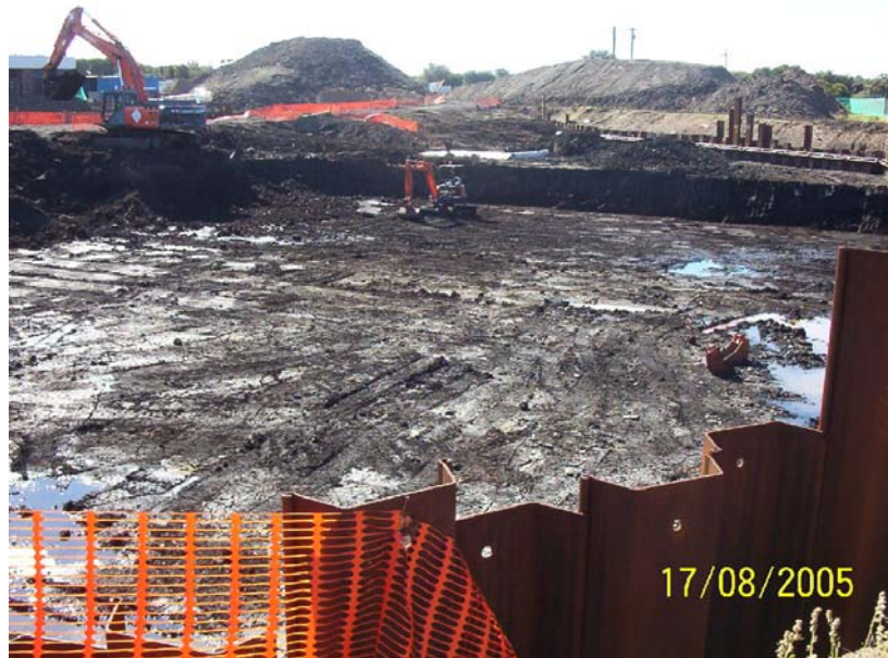
Figure 6: Approaching final excavation level.
