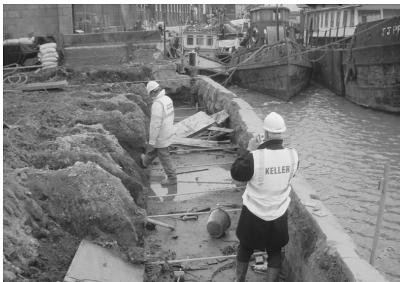
Figure 8: LCM mass gravity block behind existing quay wall at Barking, United Kingdom
