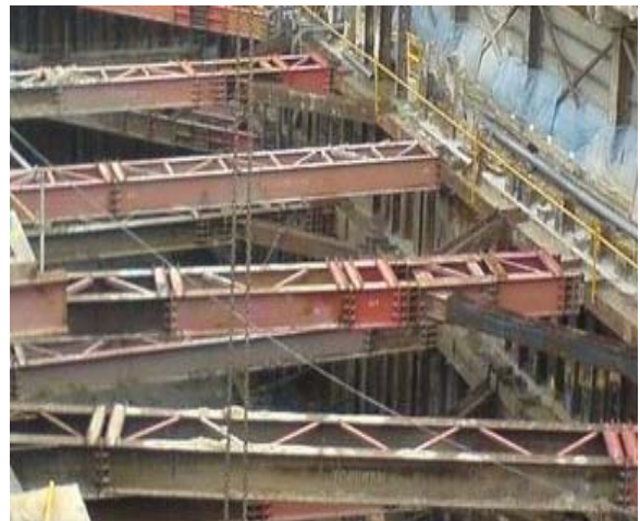
Figure 4: Laced beam girder struts.
