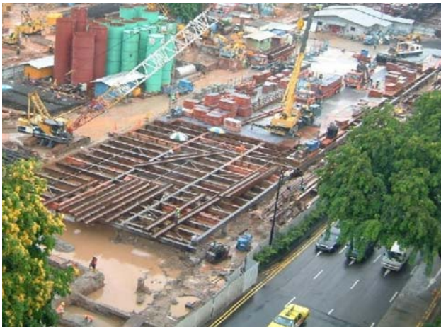
Figure 7: Steelwork construction with traffic on the right.
