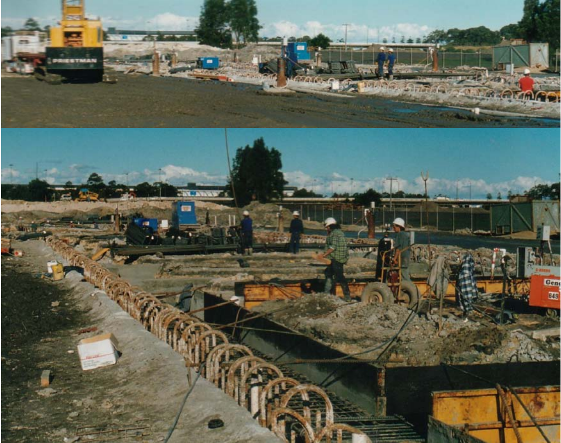
Figure 8: Dewatering excavation for New Southern Railway.
