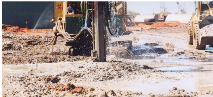
Figure 14: Ground improvement by vibrocompaction.
