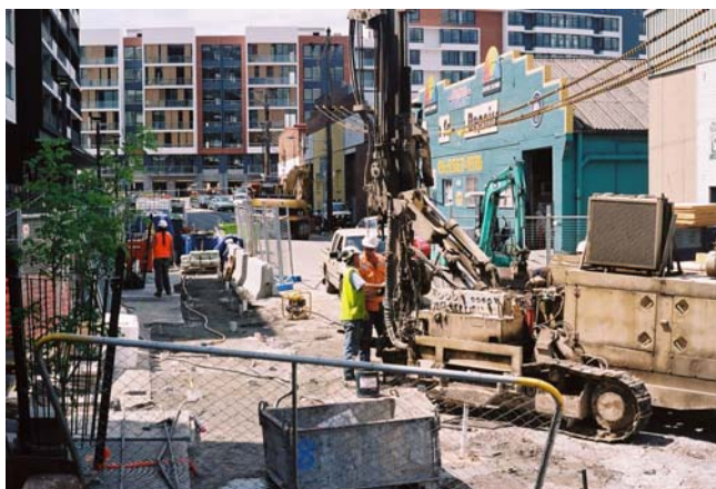
Figure 11: Ground treatment at Arncliffe.
