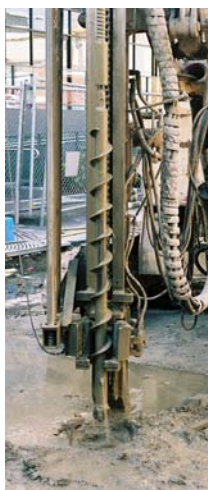
Figure 12: Grouting for manhole construction.
