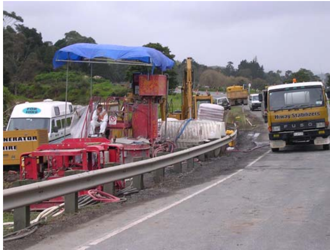
Figure 15: Treatment of Portland Landslide by Colmix.
