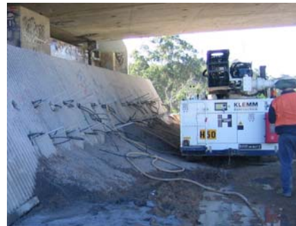
Figure 5: Soil nailing on EastLink, Melbourne and Lane Cove tunnel project, Sydney.
