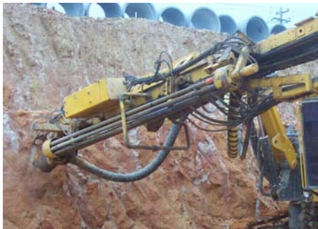
Figure 5: Soil nailing on EastLink, Melbourne and Lane Cove tunnel project, Sydney.
