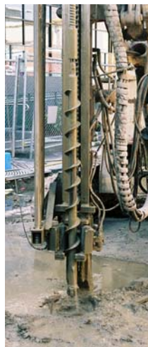
Figure 12: Grouting for manhole construction.
