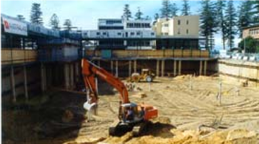
Figure 1: Densification to increase the bearing capacity and reduce settlement in marine sand.
