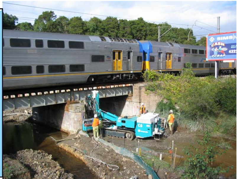
Figure 2: Previous bridge showing jet grout installation.
