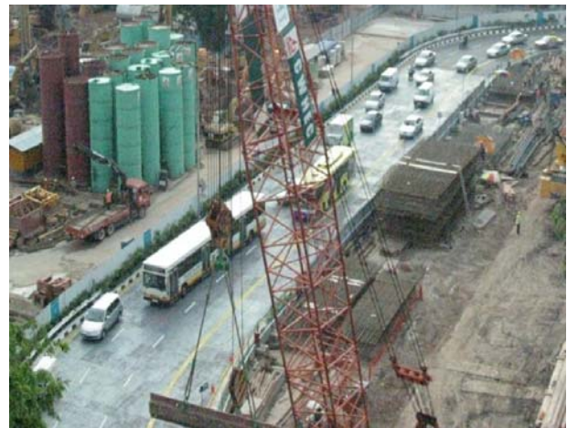
Figure 8: Traffic switched to left after steelwork completion, work proceeds on right.
