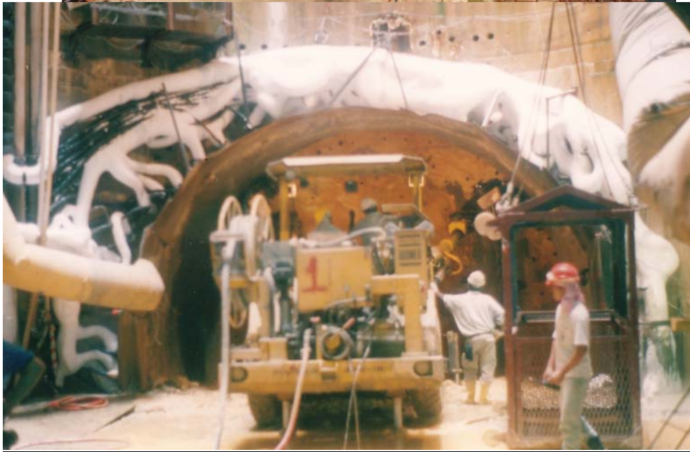
Figure 9: Freezing deep tunnel system, Singapore.
