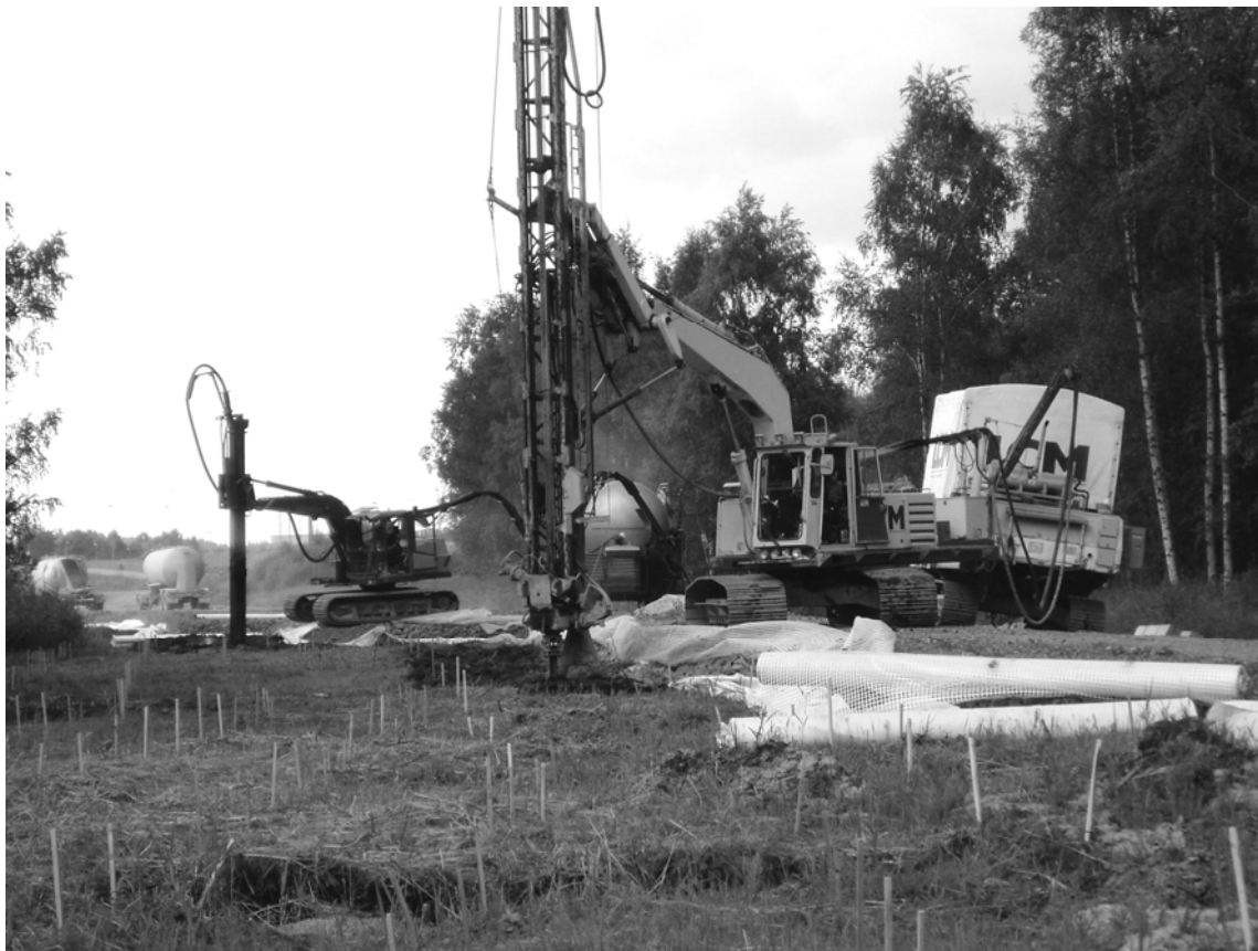
Figure 2: LCM rig and mass mixing rig at Moraberg (2003).
