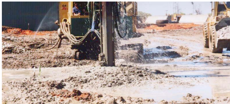
Figure 14: Ground improvement by vibrocompaction.
