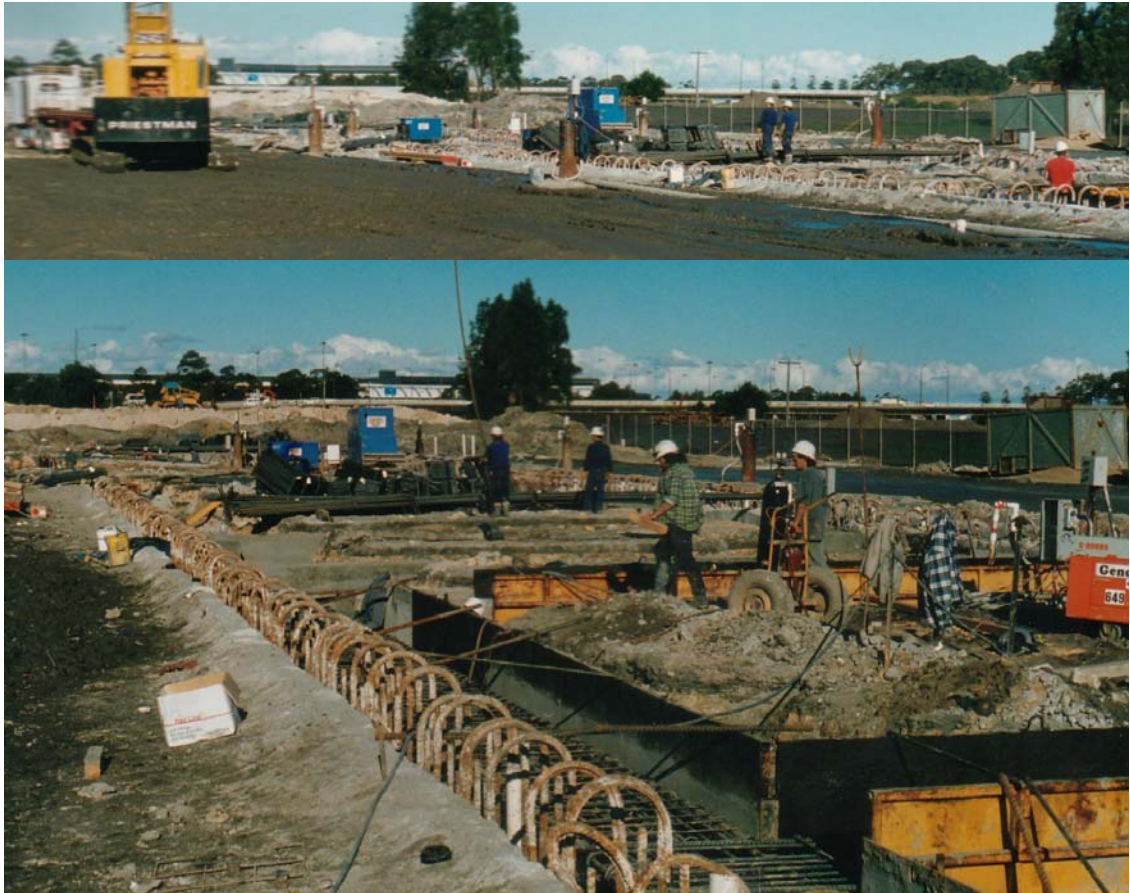
Figure 8: Dewatering excavation for New Southern Railway.
