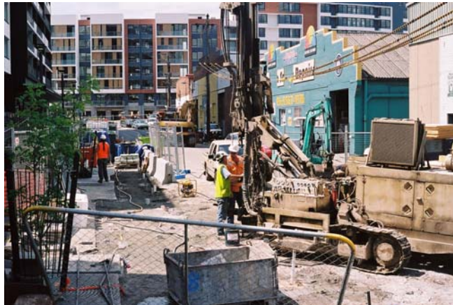
Figure 11: Ground treatment at Arncliffe.
