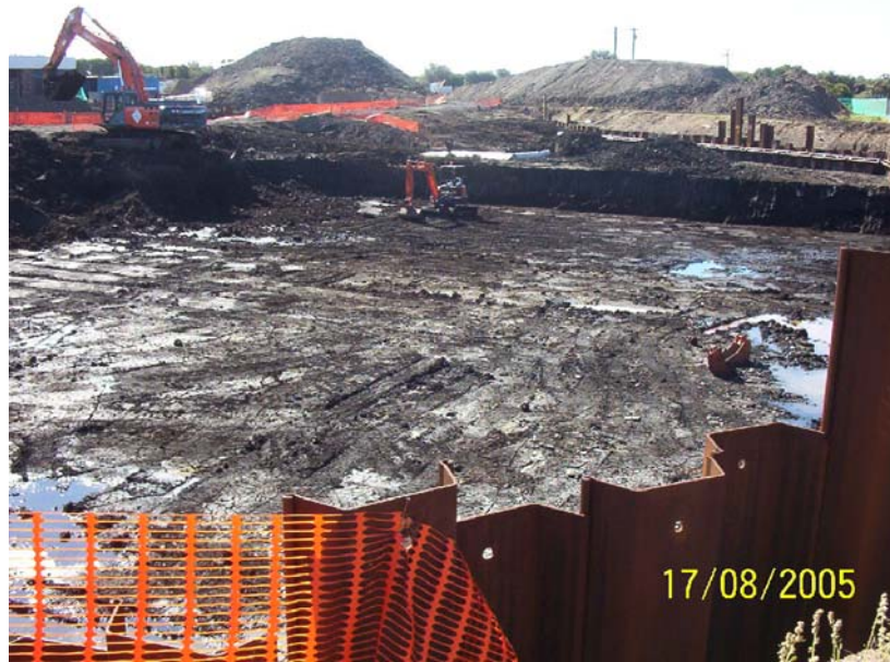
Figure 6: Approaching final excavation level.
