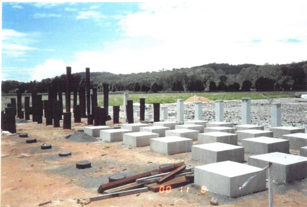
Photo 8: Constructed pile caps
