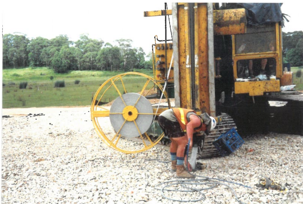
Photo 6: Close-up view of wick drainage rig
