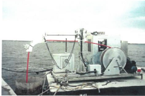
Figure 24. The SID device – ground level equipment
