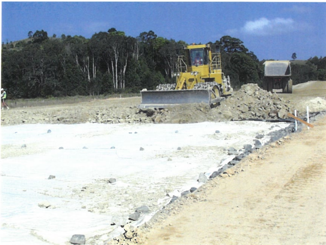
Photo 4: Placement of fill over geotextile
