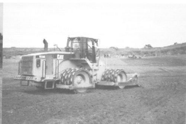
4b Fill Placement and Compaction
