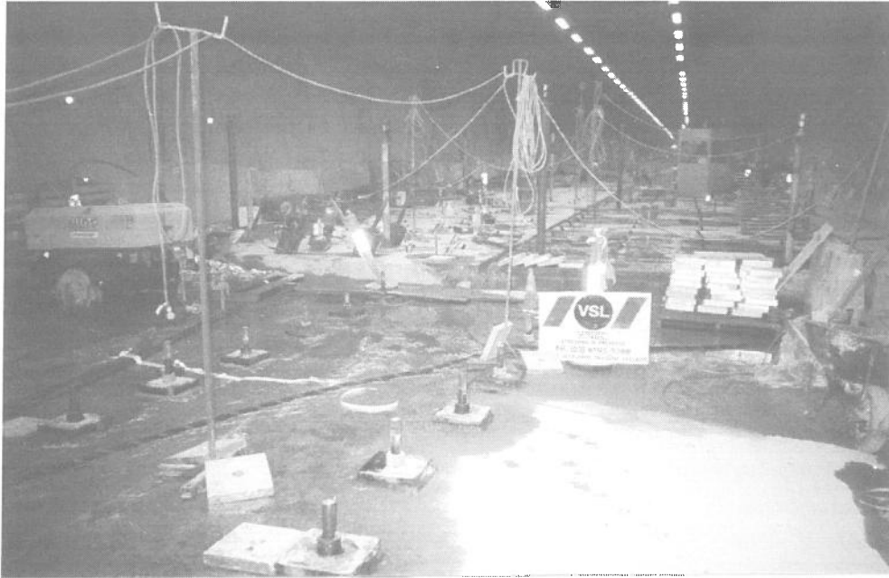
Photograph 3 – Twin anchored and multi-anchored slabs
