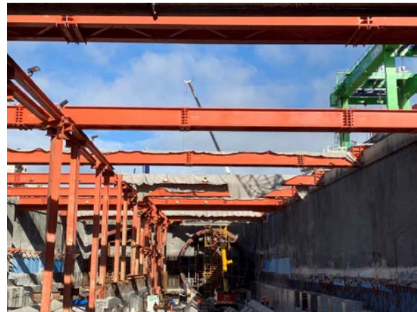
Figure 7. View of northern portal temporary strutting towards TBM headwall
