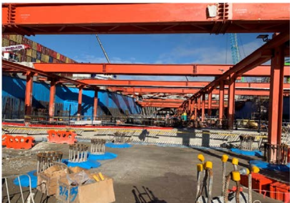
Figure 8. View of northern portal temporary strutting
