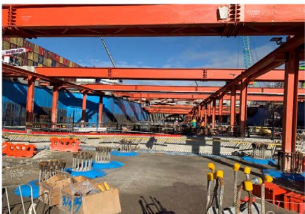
Figure 8. View of northern portal temporary strutting
