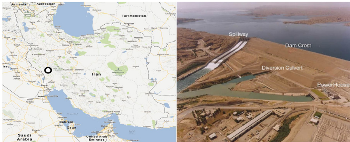
Figure 1: Location of Karkheh earth dam on Iran's map [left]; an aerial view of Karkheh earth Dam [right] (after Mirghasemi, 2006)
