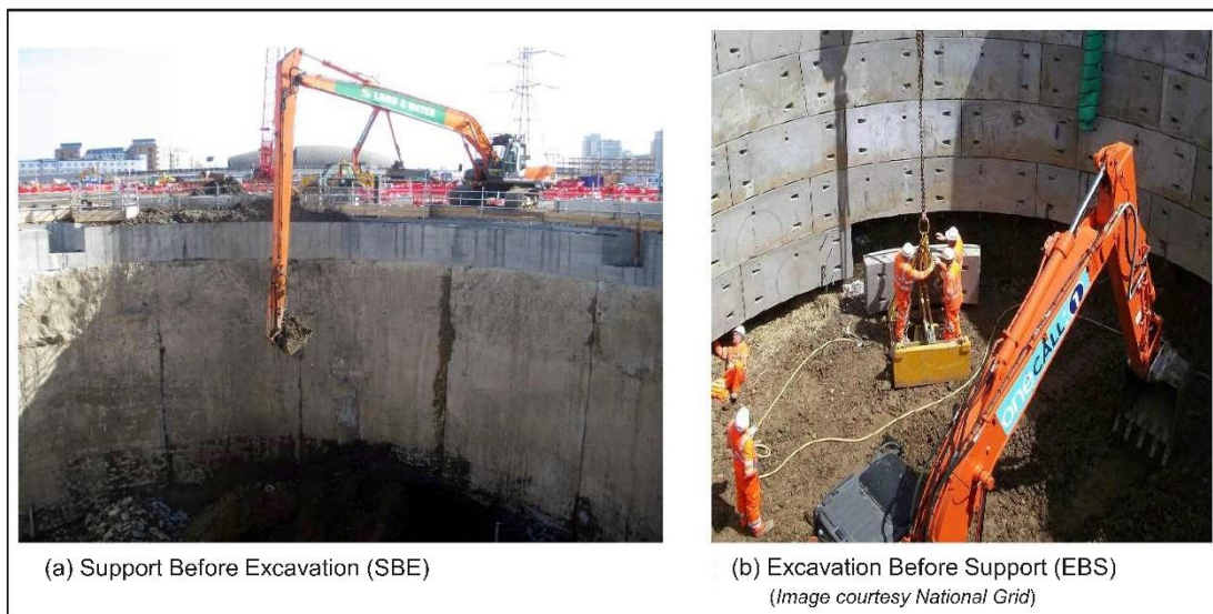
Figure 2 Two distinct shaft construction categories
