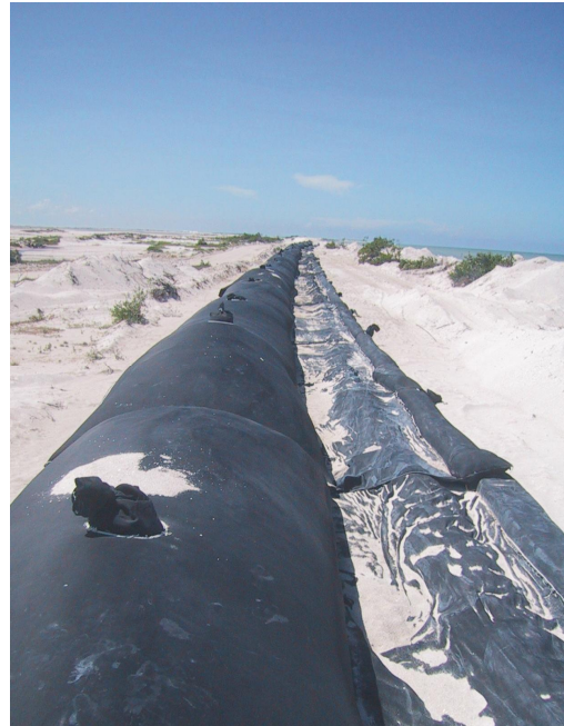
Photo 2: Geotextile with Scour Apron
