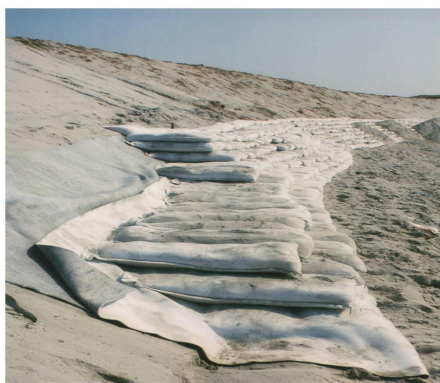
Photo 5: Geotextile Bag Placement.
