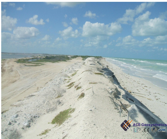
Photo 1: Geotextile Back Beach Protection.
