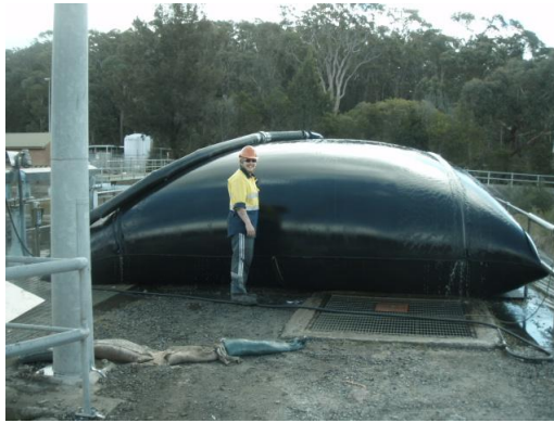
Photo 9: Geotextile tube filled.
