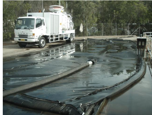
Photo 8: Filling of geotextile tube commences.
