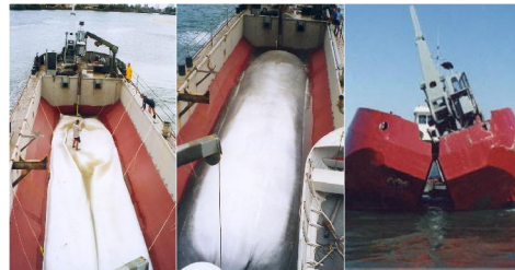
Photo 4: Geotextile Container in Barge.
