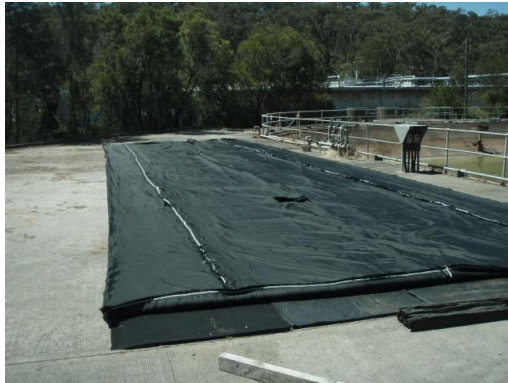
Photo 7: Positioning the geotextile tube.
