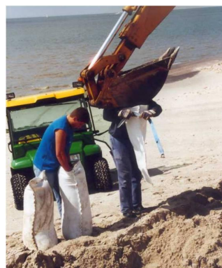
Photo 6: Filling Geotextile Bag.
