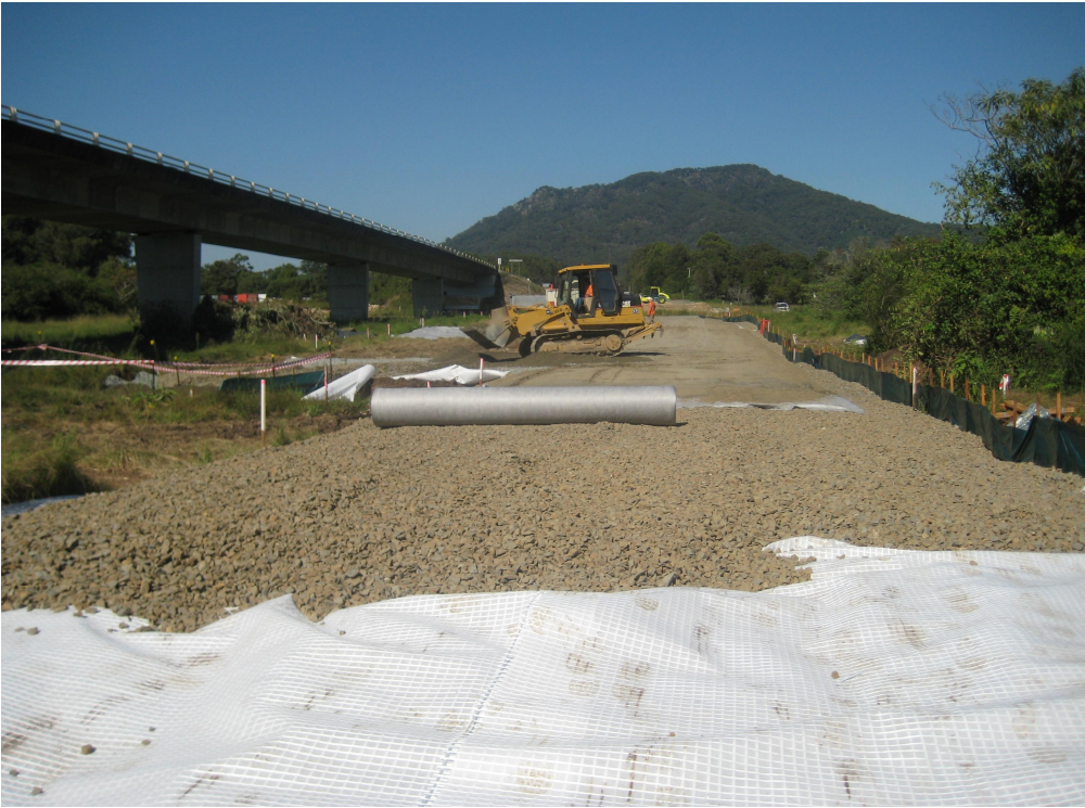
Photo 1: Installation of geosynthetic composite on site.
