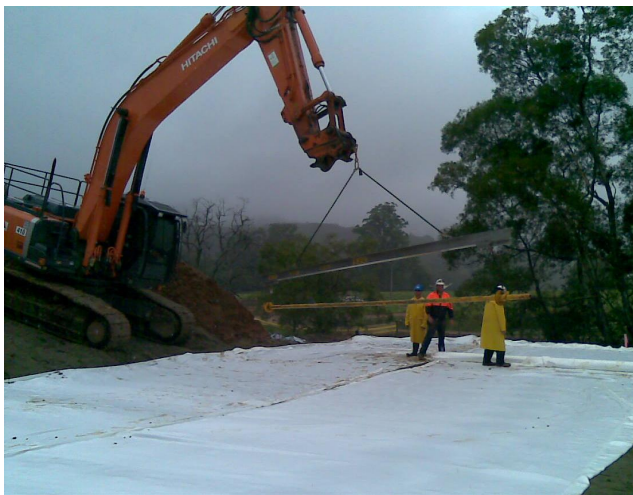
Figure 12: Placing geotextile in longitudinal direction.
