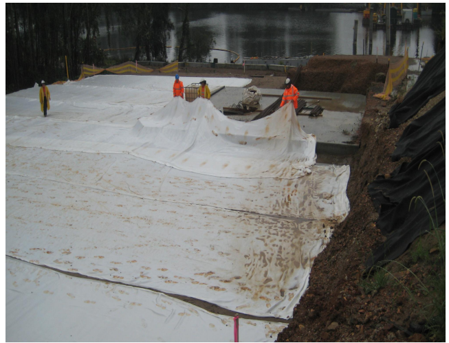
Figure 11: Placing geotextile in transverse direction.
