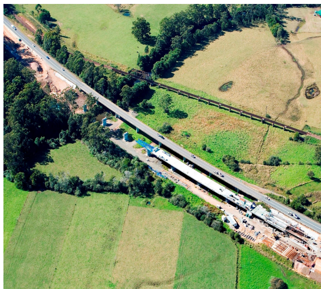
Figure 1: Existing Stewart's River bridge.
