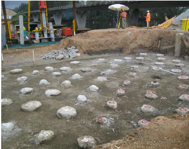
Figure 10: Installed column layout at Camden Haven River.
