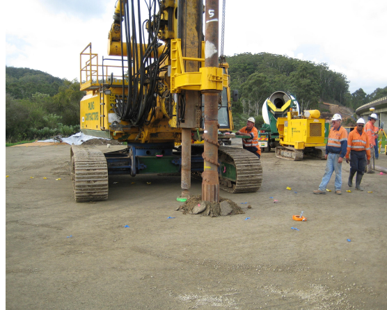
Figure 7: Column installation.
