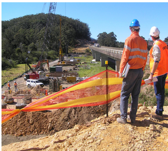
Figure 5: Construction of new Stewarts River Bridge.
