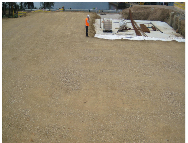
Figure 13: Completed load transfer mat showing section of concrete load transfer mat.
