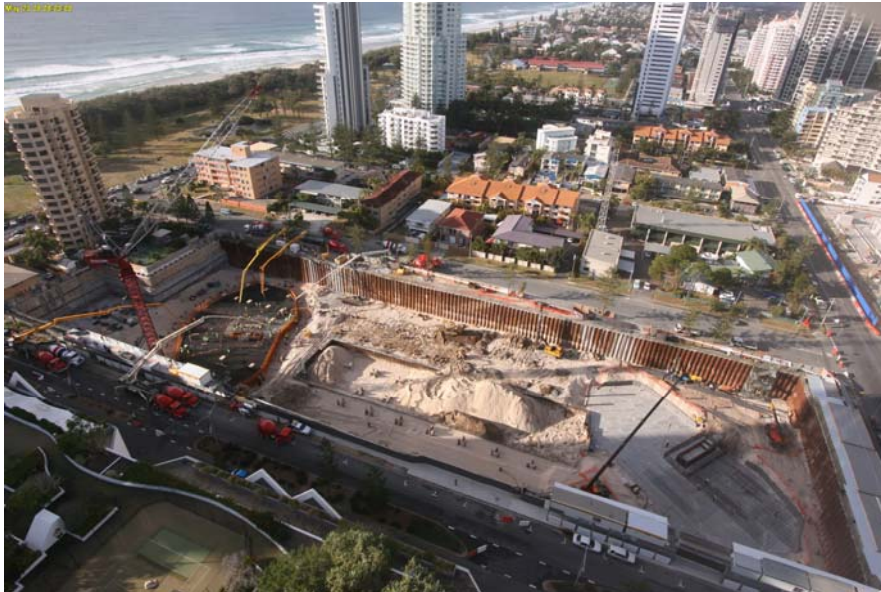
Figure 5 – Photograph of site during pouring of tower raft slab
