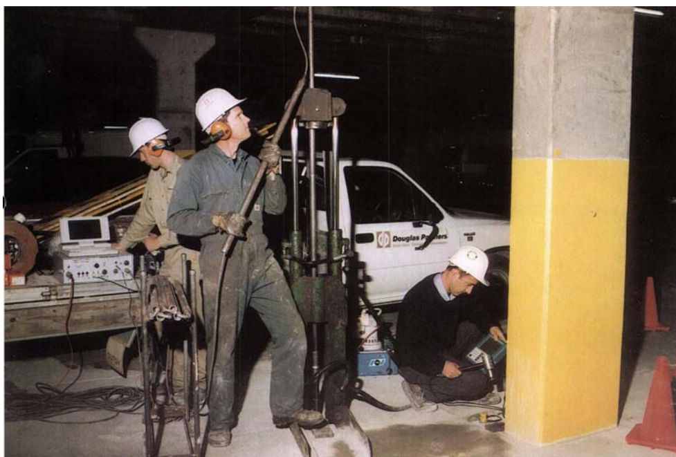
Figure 1: Portable CPT rig in operation for a building upgrade project.
