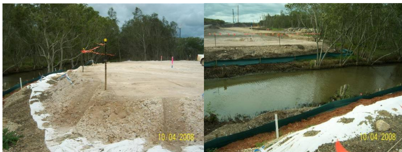
Figure 7: Polyfelt WX installed at BR25A and BR25B
