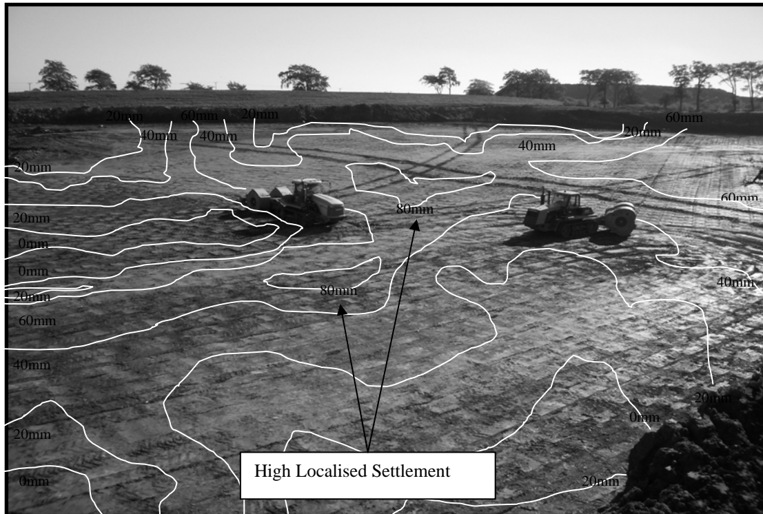
Figure 8: Plot showing Compaction Settlement over 10 Passes
