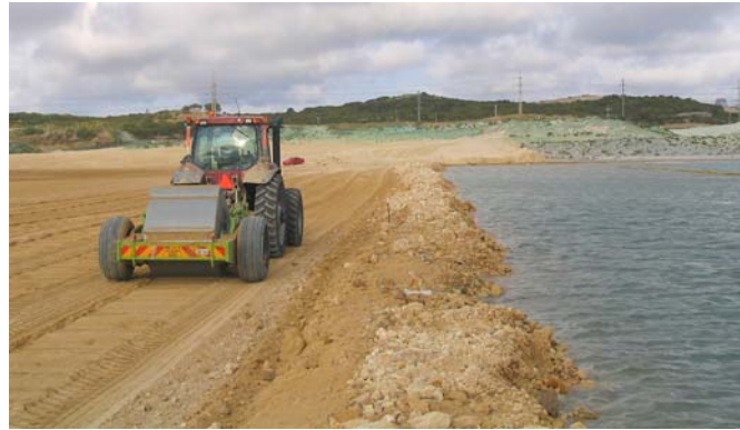
Figure 1: Impact rolling at Port Coogee, WA.
