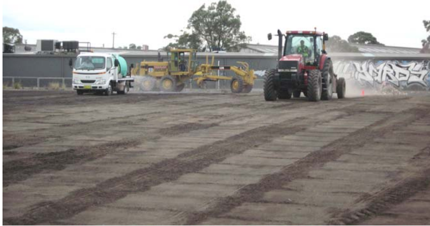
Figure 8: Trial underway on site in Sydney, NSW.
