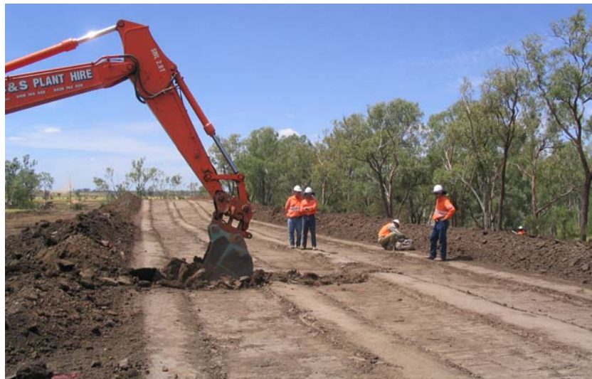
Figure 7: Trial embankment at Curragh North, Queensland.
