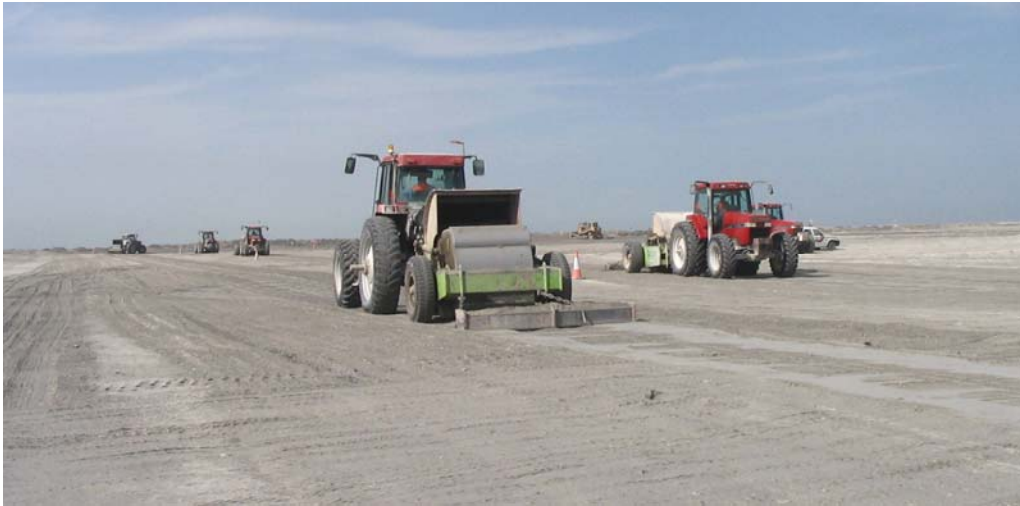
Figure 3: Impact rolling at the NDIA project, Qatar.
