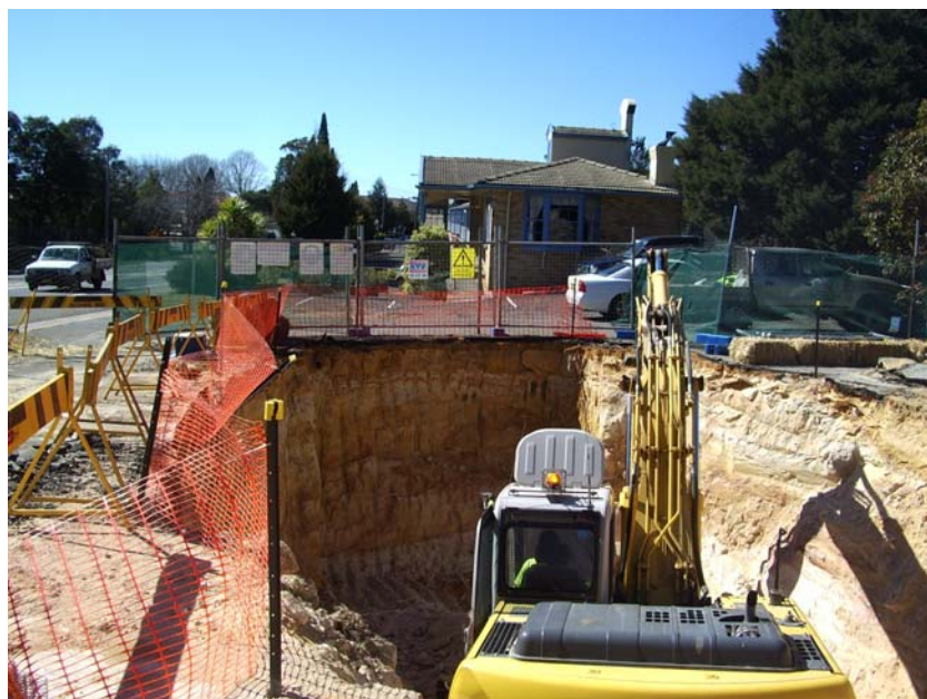
Figure 1: Underground storage tank excavation in road verge, Great Western Highway upgrade.
