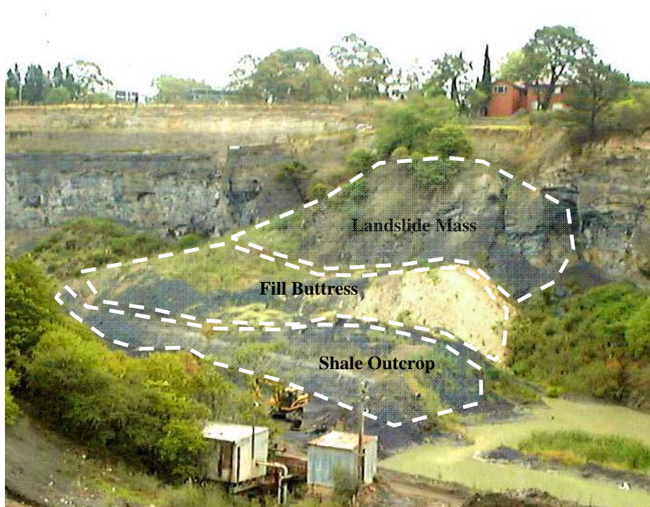
Figure 4: View of slip looking north west.
