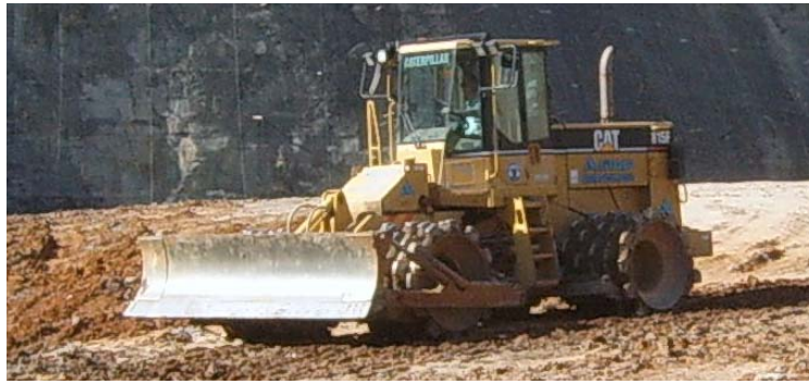
Figure 13: Remote controlled CAT815.
