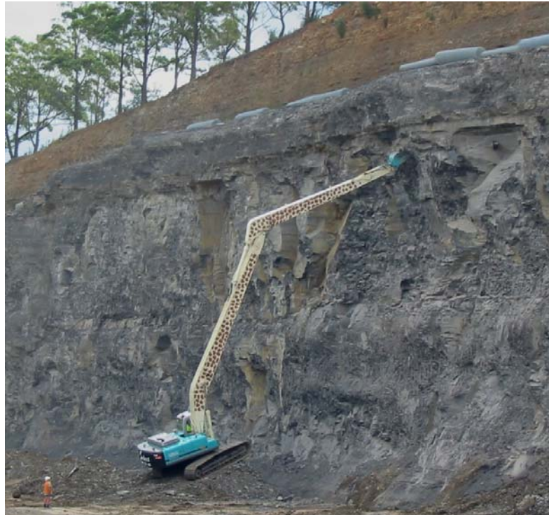
Figure 5: Scaling using long reach excavator.
