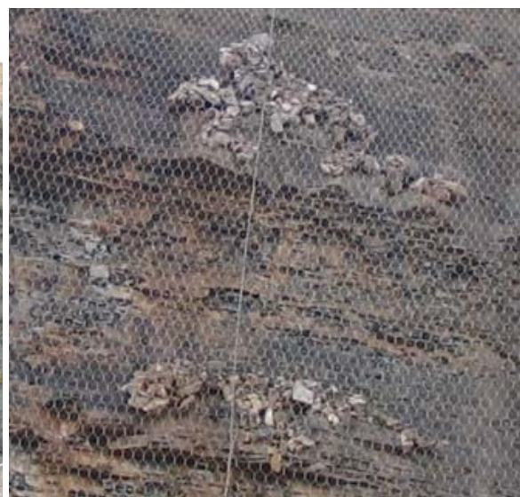
Figure 7: Rock fall captured by mesh.
