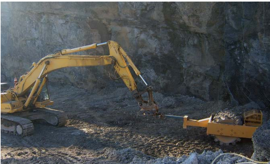
Figure 11: Modified towed roller attached to excavator.
