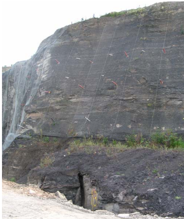
Figure 18: Remediated landslide with remaining slip material left at base.
