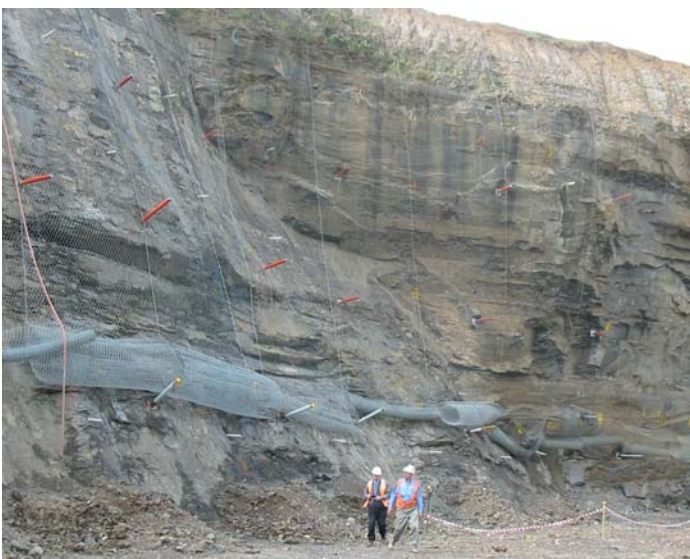
Figure 6: Batter mesh installed on north pit wall.
