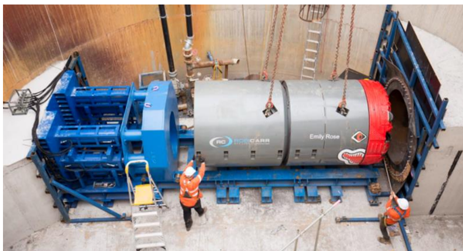
Figure 7: Microtunnel installation in caisson
