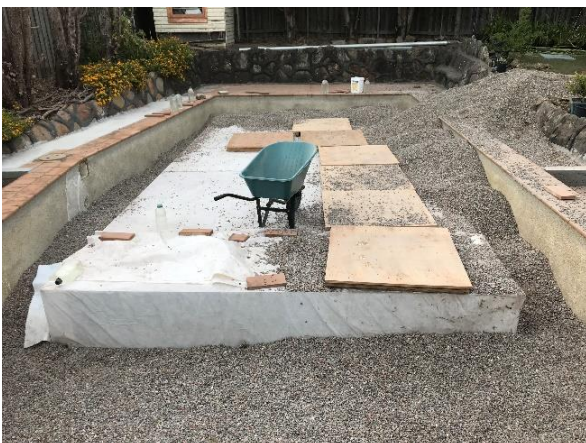
Figure 11: Backfilling around double units
