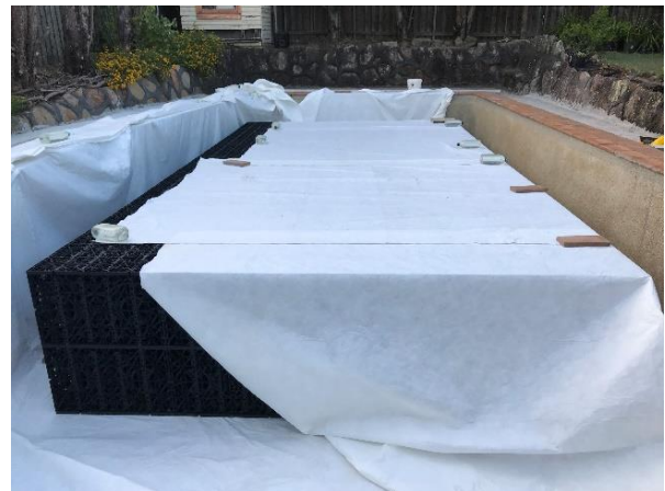
Figure 10: Double units and geofabric wrap
