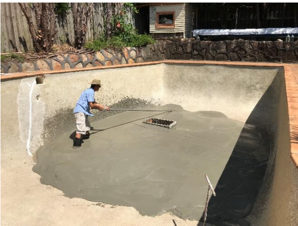
Figure 9: Placement of liquifill levelling layer
