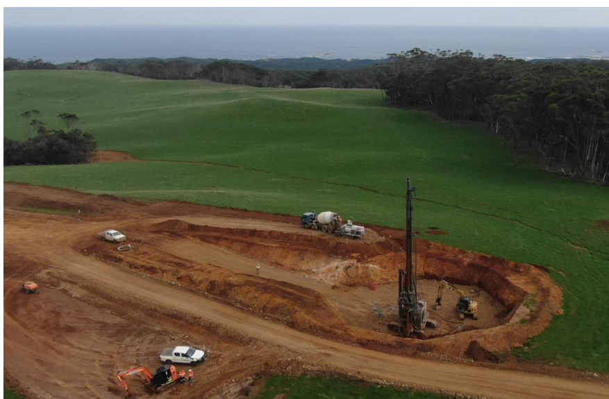
Figure 5: Installation of CMC at Granville Harbour Wind Farm
