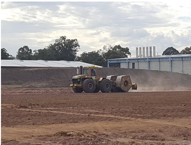
Figure 3: Tractor and pentagonal drum used
