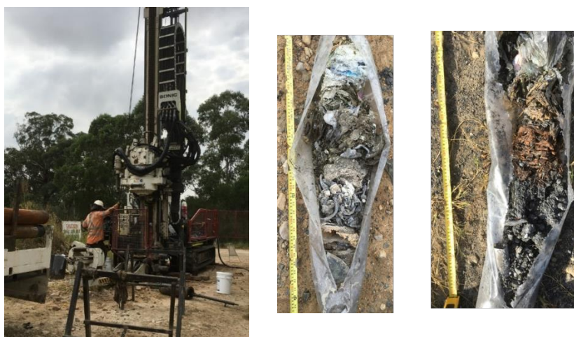
Figure 1: Typical sonic drilling and MSW samples recovered during sonic drilling
