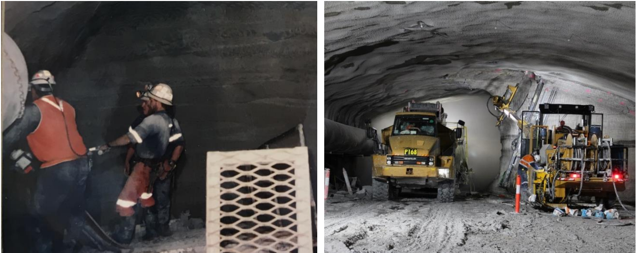
Figure 4: Hand-installed (left) and remote bolting (right)
