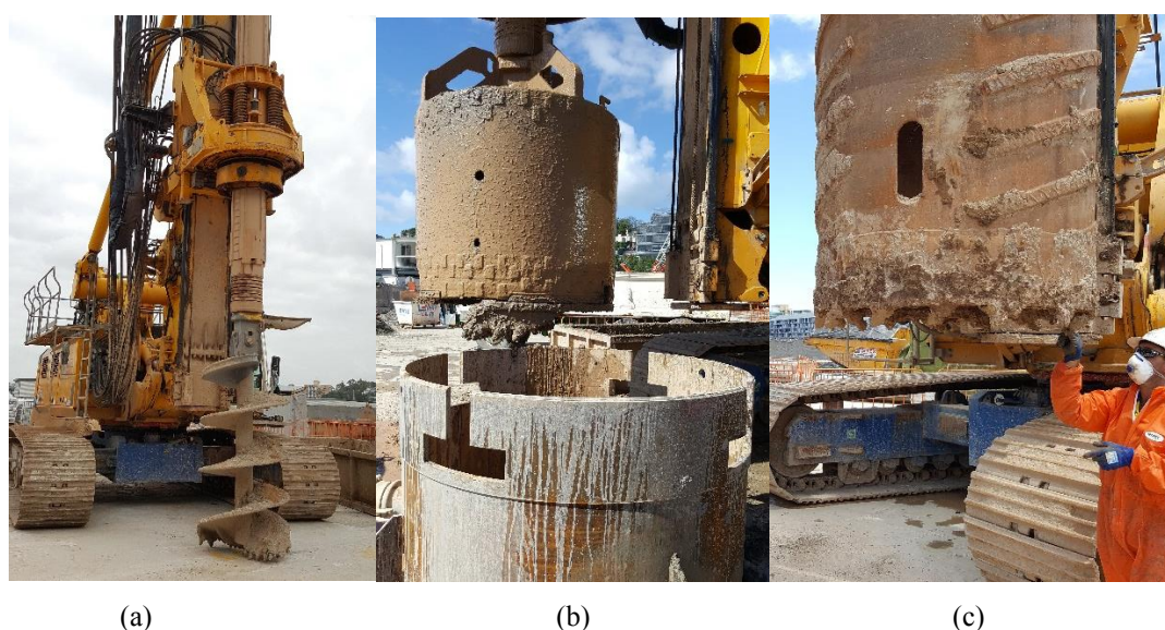
Figure 8: (a) Auger, (b) drilling bucket and (c) core barrel
