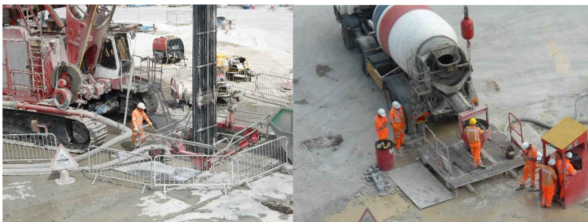
Figure 7: Edge protection barriers fixed to guide walls (left) and panel covers during concreting (right)
