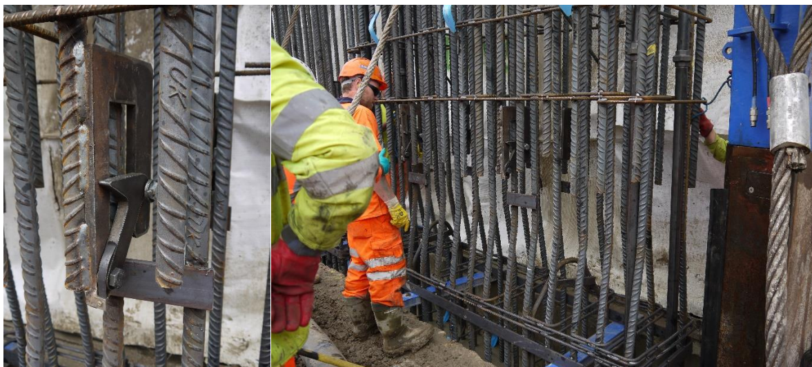
Figure 8: Superlatch cage splicing system
