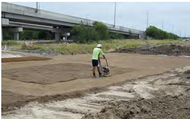
(e) Earth fill cover placement
