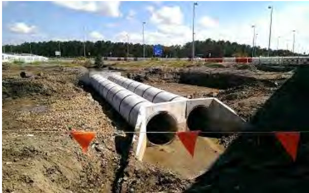
(a) Excavation to base level
