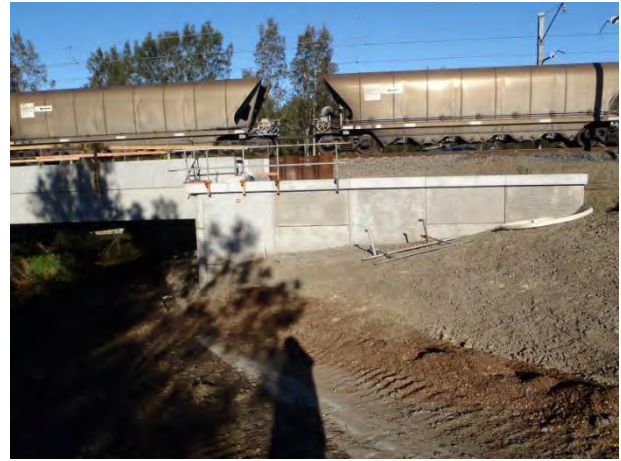
Photo 5: Completed Trapezoidal-RSW at Wyoming Creek
