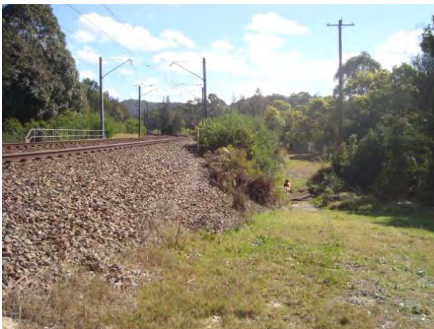
Photo 2: Pre-construction – Site of proposed rail embankment widening
