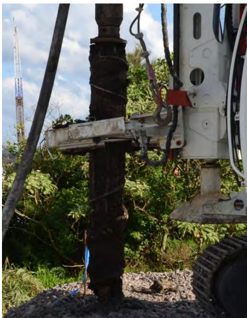
Figure 1: CMC auger (Gerringong Upgrade project, 2013)
