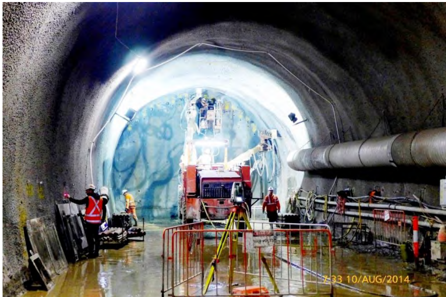
Figure 6: Canopy tube installation with shotcrete lining in foreground.
