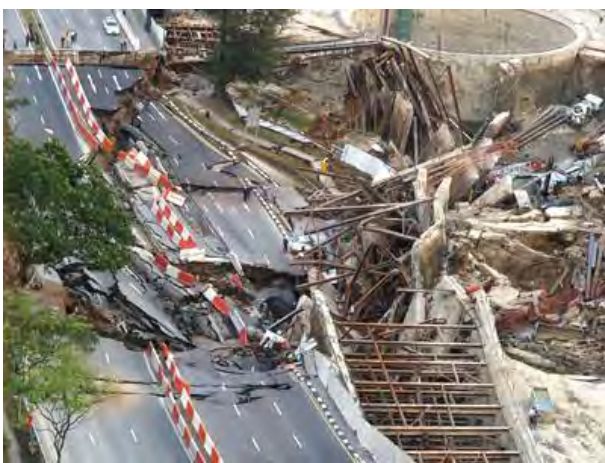
Figure 8: Post-failure photo of Nicoll Highway Collapse.
