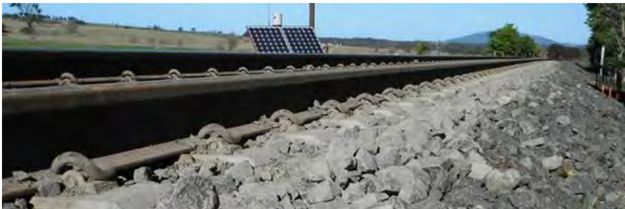
Figure 14: Track profile after retamping.
