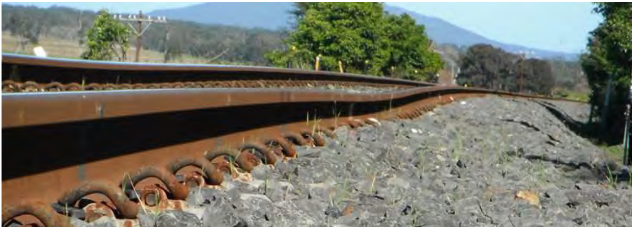
Figure 13: Track profile before retamping.
