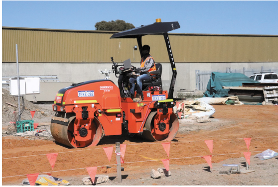
Figure 10. A double-drum roller instrumented with SPARC IC kit (Site: SPARC test pit in Notting Hill, Victoria)
