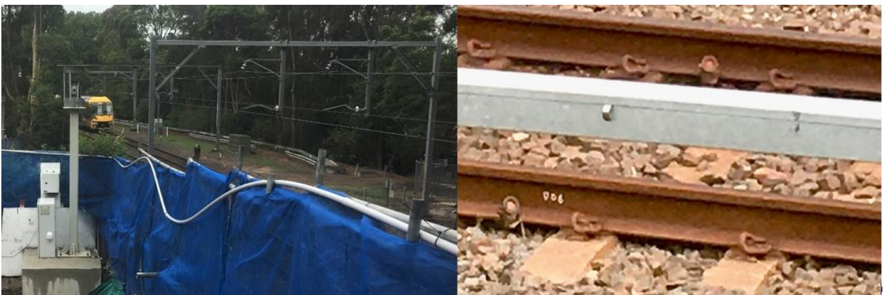
Figure 16: View along railway showing automated remote monitoring detail
