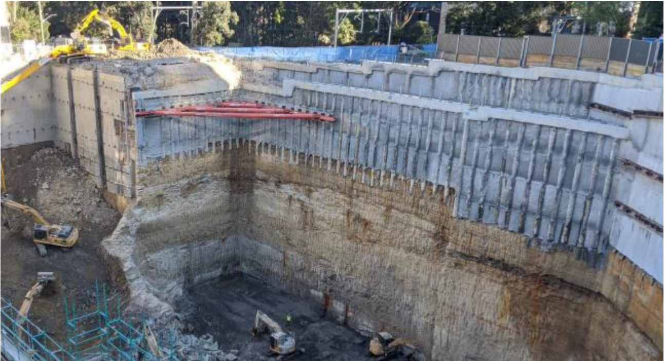
Figure 6: Excavation support along Sydney Trains (west) boundary
