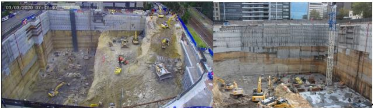
Figure 10: Bulk excavation works - view to south and north
