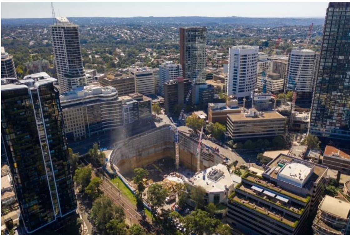
Figure 2: Aerial view perspective of the excavation
