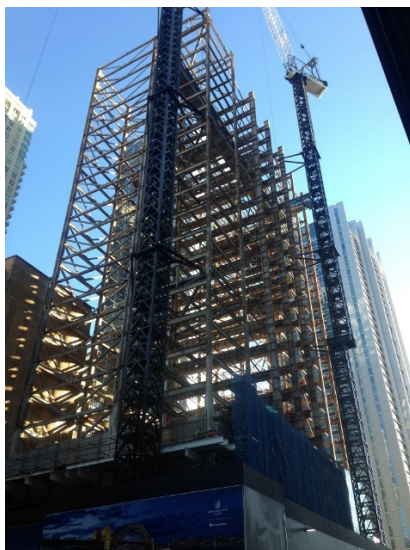
Figure 6: Old steel frame retained
