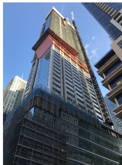
Figure 7: New building (at ~80%)
