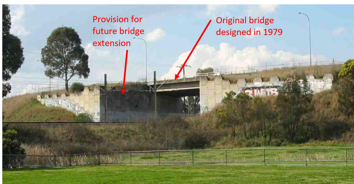
Figure 4: Bridge abutment in 2011 – view 1
