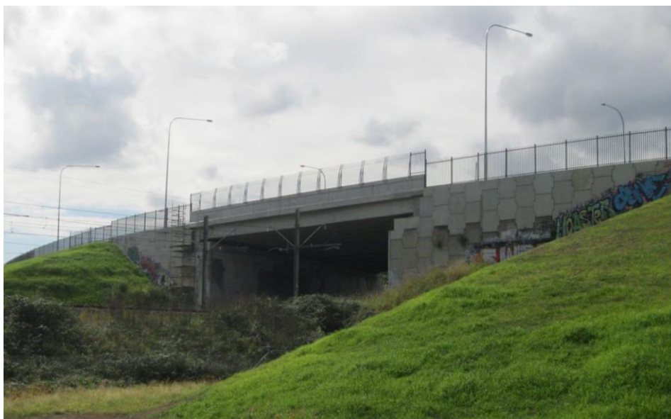
Figure 10: New reinforced earth walls and bridge, completed in 2013
