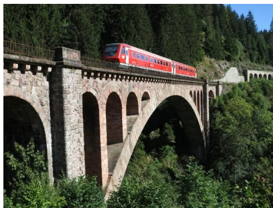
Figure 2: Gutach Rail Bridge built in 1900 with a main span of 64m (Structurae, 2020).
